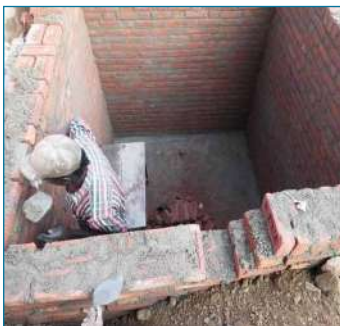
GGMS, Unchehra toilet repair
